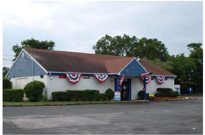
Location 2: View looking southwest towards commercial property north of LIRR and west side of CR 31 in B-3 District
