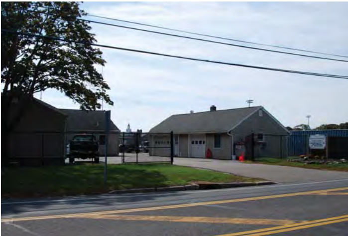
Location 34: View looking south towards school services building on south side of CR 80 and west of CR 31 in B-2 District
