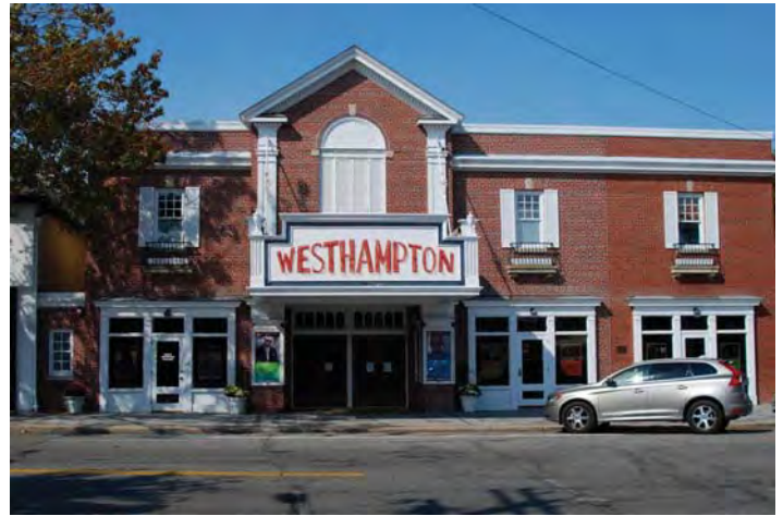
Location 20: View looking north towards Westhampton Performing Arts Center along Main St. in B-1 District
