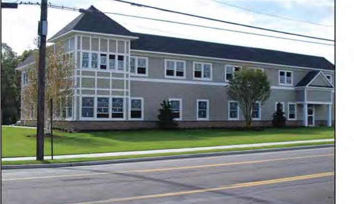
1. New building that could provide diverse business.
