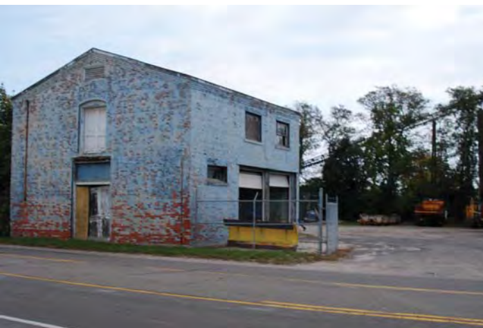
Location 5: View looking east towards Town DPW yard south of LIRR and east side of CR 31 in B-3 District
