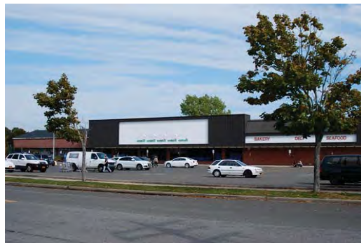
Location 41: View looking east toward vacant grocery retail along Sunset Ave. in B-1 District
