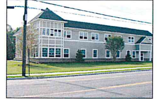
1. New building that could provide diverse business.
