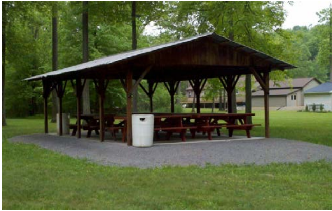
Shelter 1-near NEW restrooms
