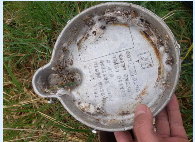
Insect infestation under a standard well cap (photo courtesy of Clark Beebe, MWON volunteer, Bradford County).
