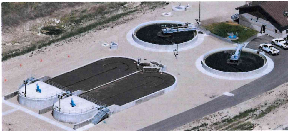
FIGURE 4-8: OXIDATION DITCHES AND SECONDARY CLARIFIERS
