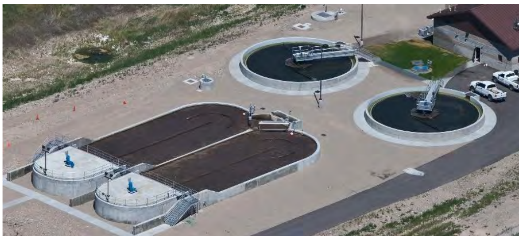
FIGURE 4-8: OXIDATION DITCHES AND SECONDARY CLERIFIERS
