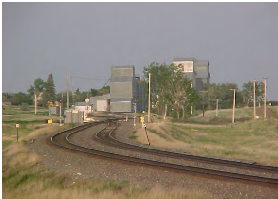
Figure 1-5: The railroad has connected communities within the county for decades.
