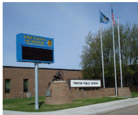
Figure 5-4: Retaining quality schools is important to the community
