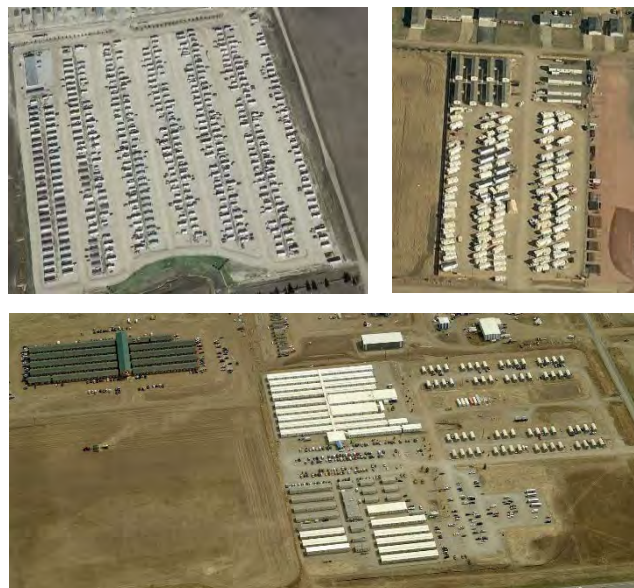
Workforce lodging facilities in Tioga (top right) and Williston (top left, bottom).
