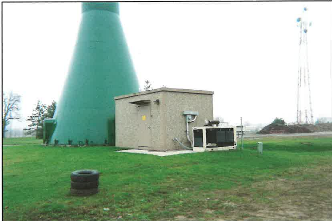
PHOTO NO. 16: Water tower adjoining the property to the east.
