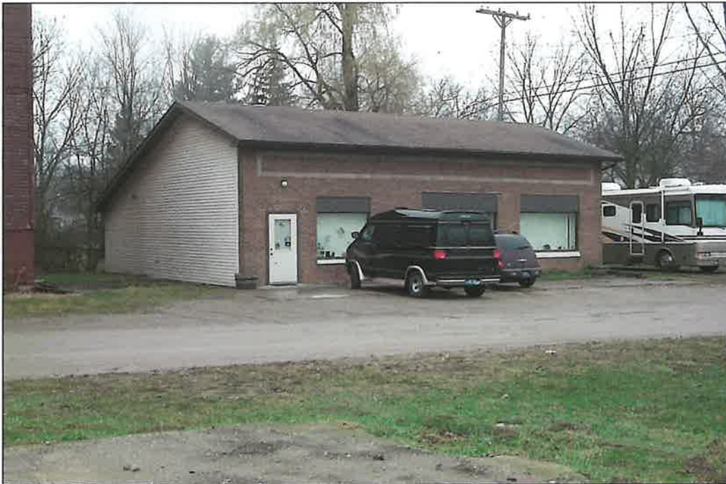
PHOTO NO. 18: A building adjoining the property to the west.
