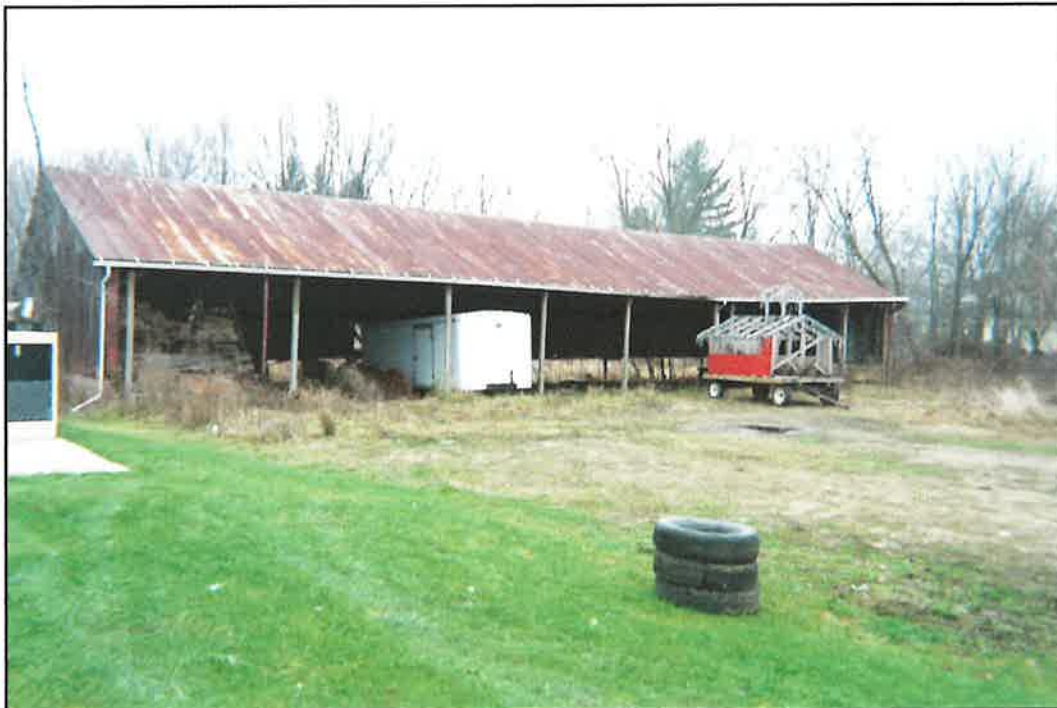
PHOTO NO. 2: Storage shed located south of the Elevator building.
