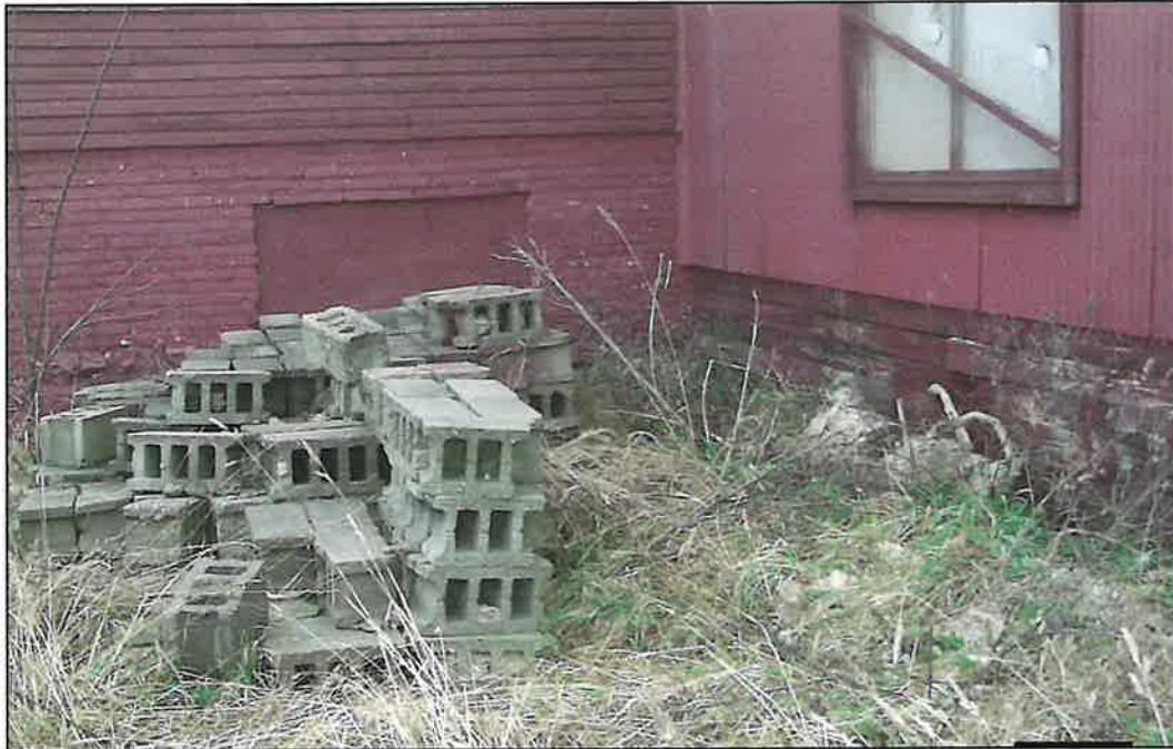
PHOTO NO. 15: Pile of discarded bricks located on the south side of the Elevator building.
