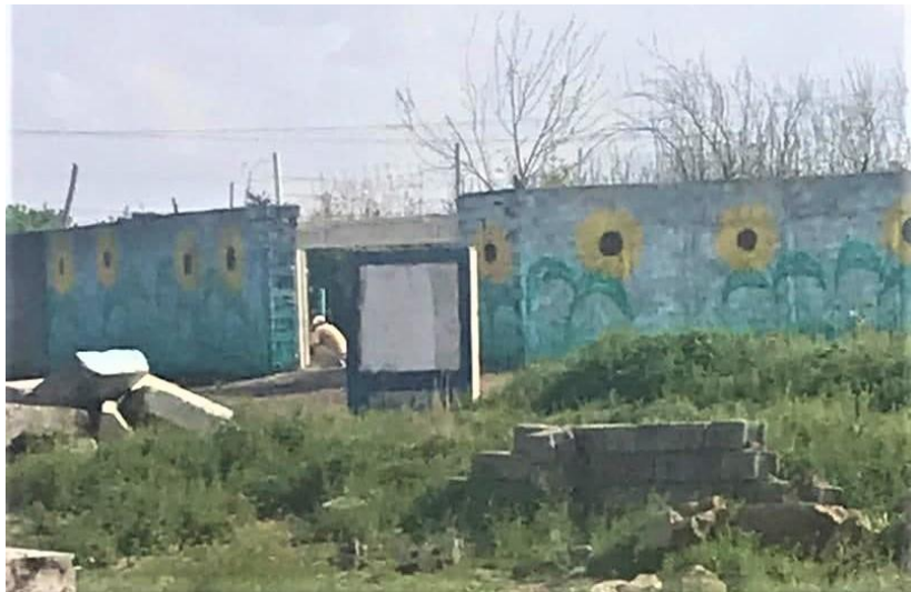
Figure 6-11. The same wall as in Figure 6-10 is painted over. Photo was taken seventy days after the incident.
