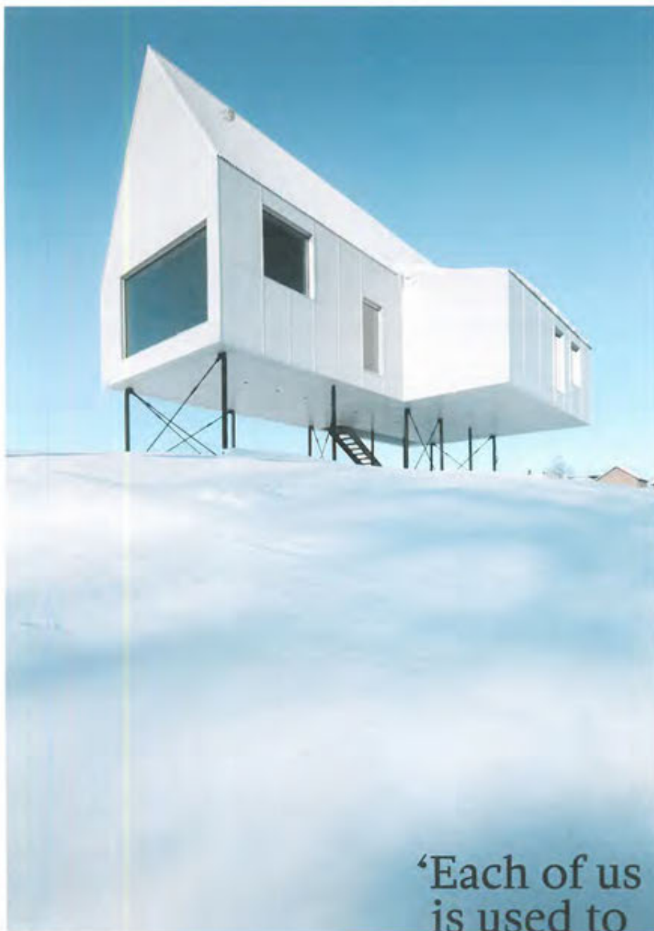
High House rests on stilts – an architectural solution typically found in warm climates and flood zones – that protect occupants from the snow below.
