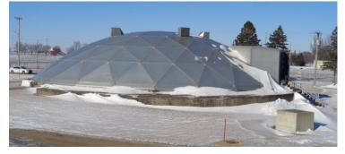
1995. An extensive upgrade to the WWTP is tentatively scheduled for 2026. The WWTP is an activated sludge process with trickling filter, clarifiers, two lift stations, ultraviolet disinfection, grit chamber and containment pond. The average daily flow to the plant is 250,000 gallons and the plant has a maximum design capacity of 1,400,000 gallons.
