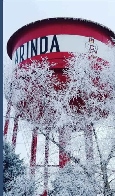
Clarinda operates a water and wastewater utility.
