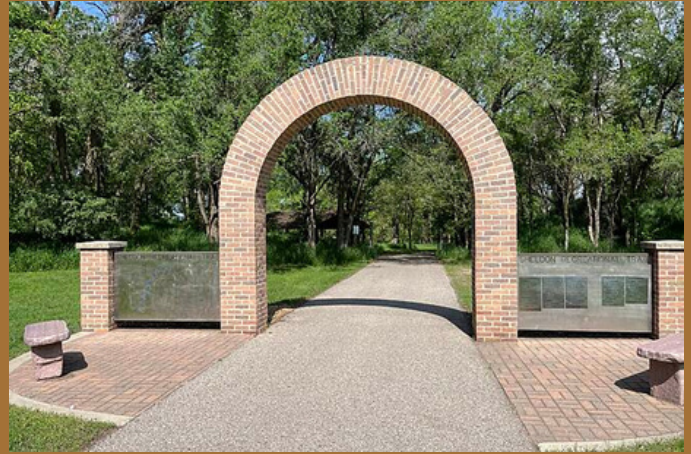
The brick trailhead archway located in Hills Park hosts donor plaques for the Sheldon Recreational Trail Head.
