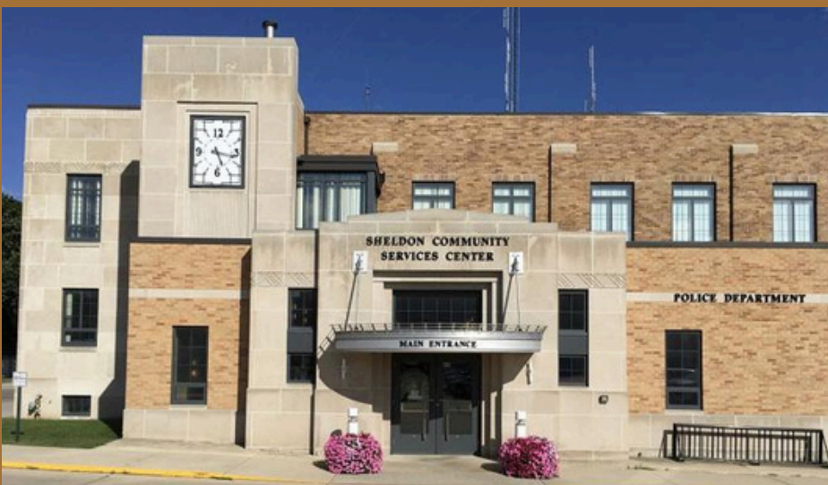
Sheldon's City Hall is located in the Sheldon Community Services Center, opened in 1939. This iconic Art Deco structure houses city offices, Police, Fire, and Community Ambulance Team, as well as the Sheldon Chamber and Development Corporation.
