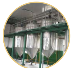
EDIBLE OIL FACILITY
