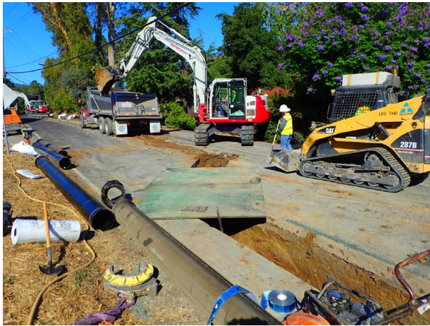
Installation of 12" ductile iron pipe along Taaffe Road.
