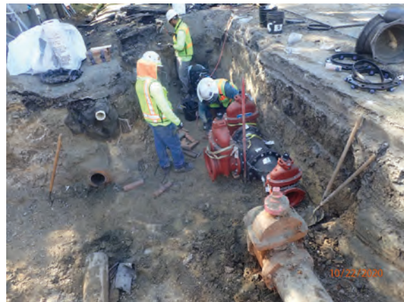
Installation of a 12" 3-valve set along Elena Road.
