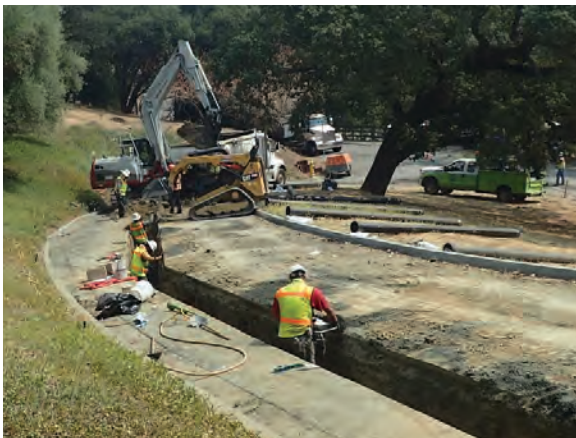
Installation of 8" ductile iron pipe along Old Snakey Road.
