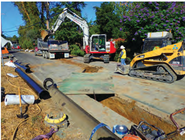
Installation of 12" ductile iron pipe along Taaffe Road.
