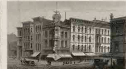
CORNER GEARY AND KEARNY STREET.
