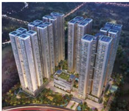
Sattva LakeRidge, Kokapet, Hyderabad
