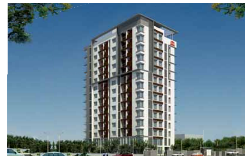
KG Chandra Vista (Semmenchery, OMR)
