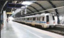
ADJACENT TO UPCOMING METRO STATION
