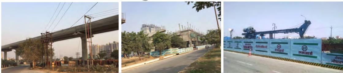
Noida-Greater Noida Metro Work in progress
