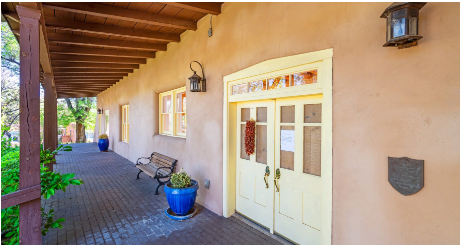
PORTAL ENTRANCE · DOUBLE DOORS ON PASEO DE PERALTA
