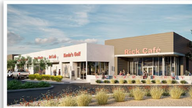
Multi-tenant Retail (Under Construction)
