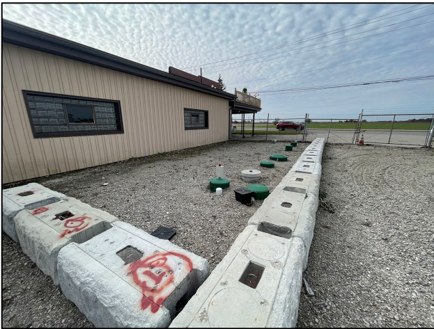
Recently updated septic system
