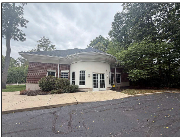
Side conference room entrance
