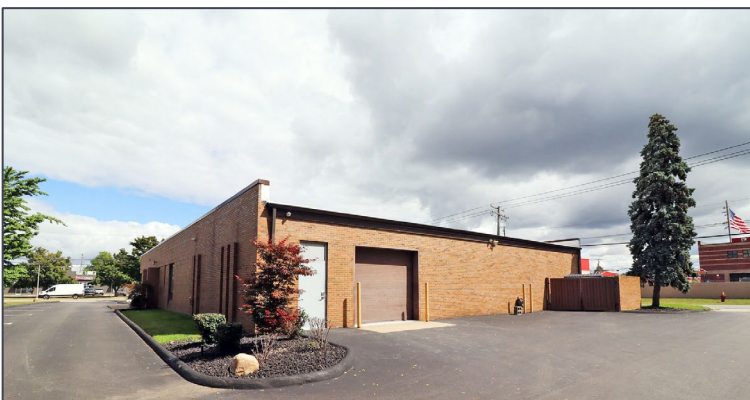
Two curb cuts. Newly paved and striped parking lot.
