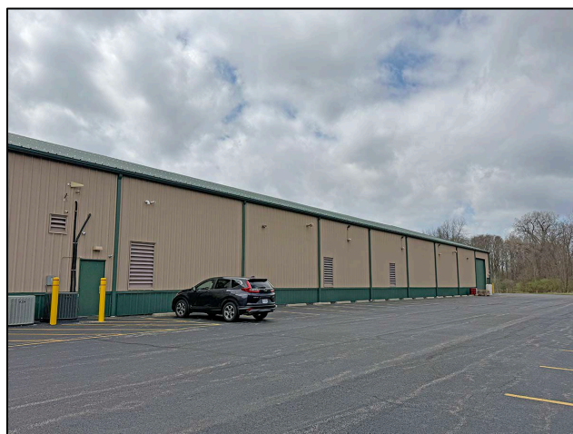
North side of property
