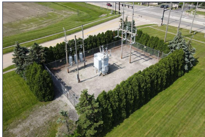
7.5/10.5 MVA 138 KVA Substation
