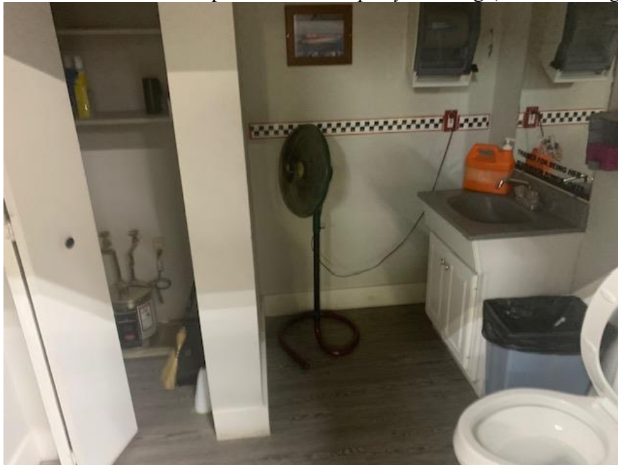
Photo 10. View of restroom inside shop area of the Property building
