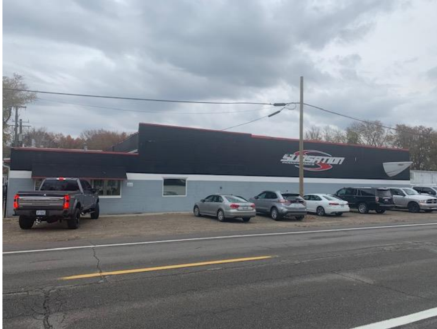
Photo 1. View of the front (south side) of the Property building
