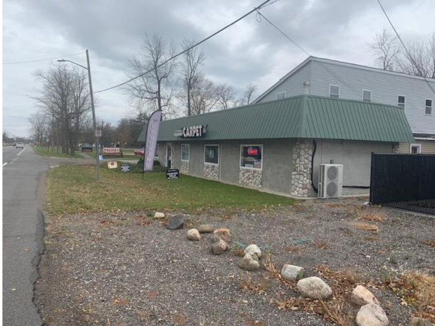
Photo 35. View of nearby commercial property (Custom Floor Covering ó 4682 Pointe Tremble Rd.) west of the Property
