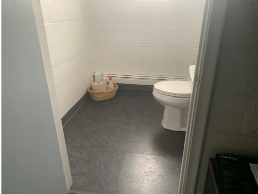
Photo 3. View of restroom inside office area of the Property building (no floor drains)
