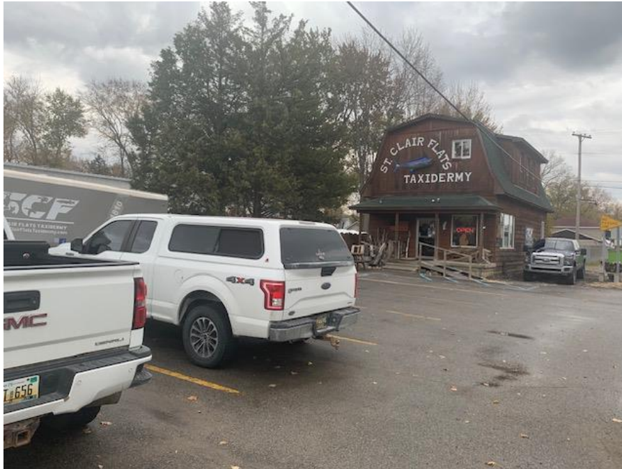
Photo 31. View of commercial property (St. Clair Flats Taxidermy -09566 Pointe Tremble Rd.) adjoining to the east-southeast of the Property
