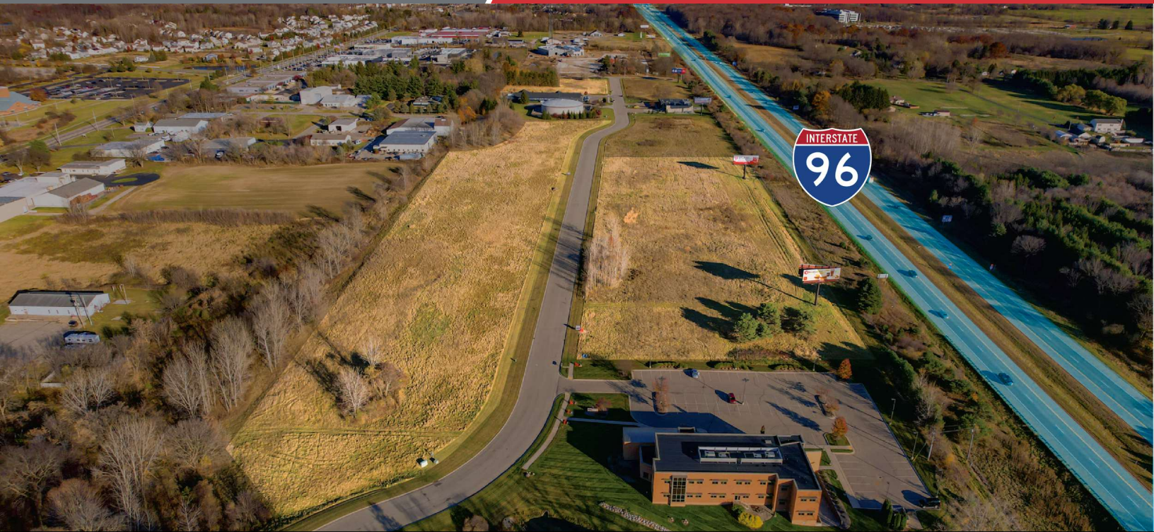
West Facing Aerial
