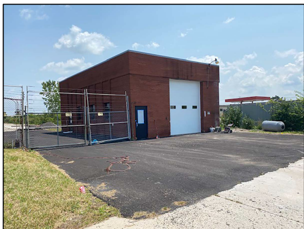
Drive in garage with 14' door
