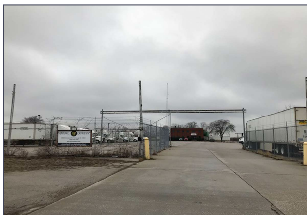
Front entry gates
