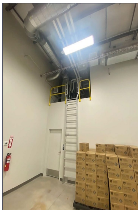
Access to HVAC
