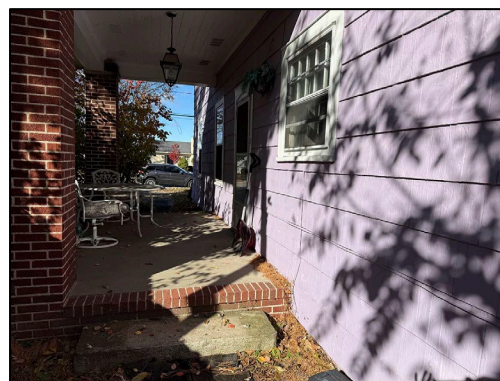
West side entry
