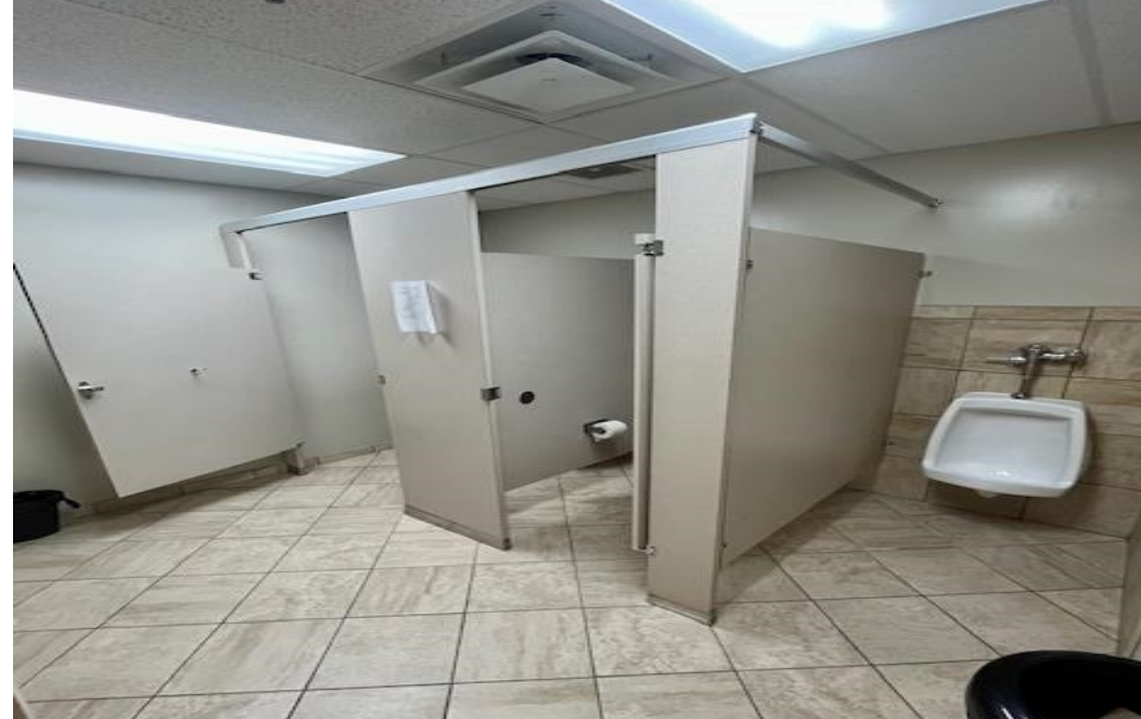
1st Floor Restroom
