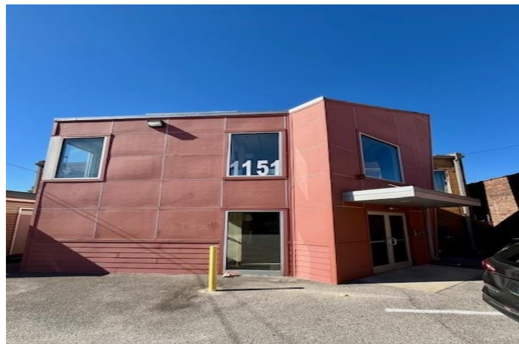
Parking Lot Entrance
