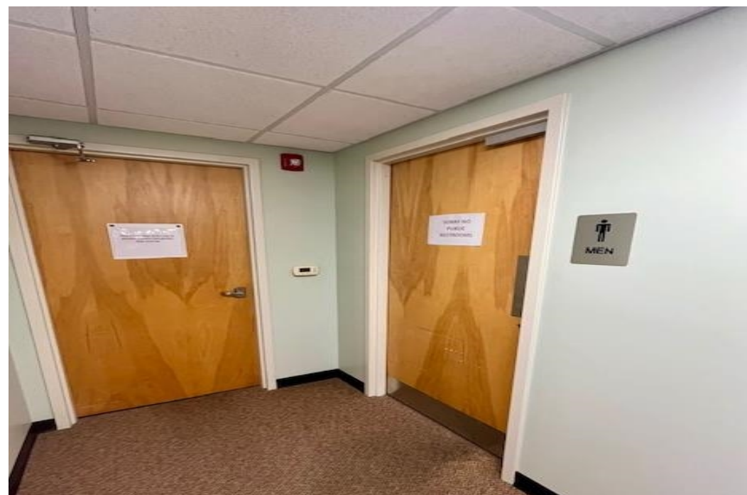
1st Floor Restrooms
