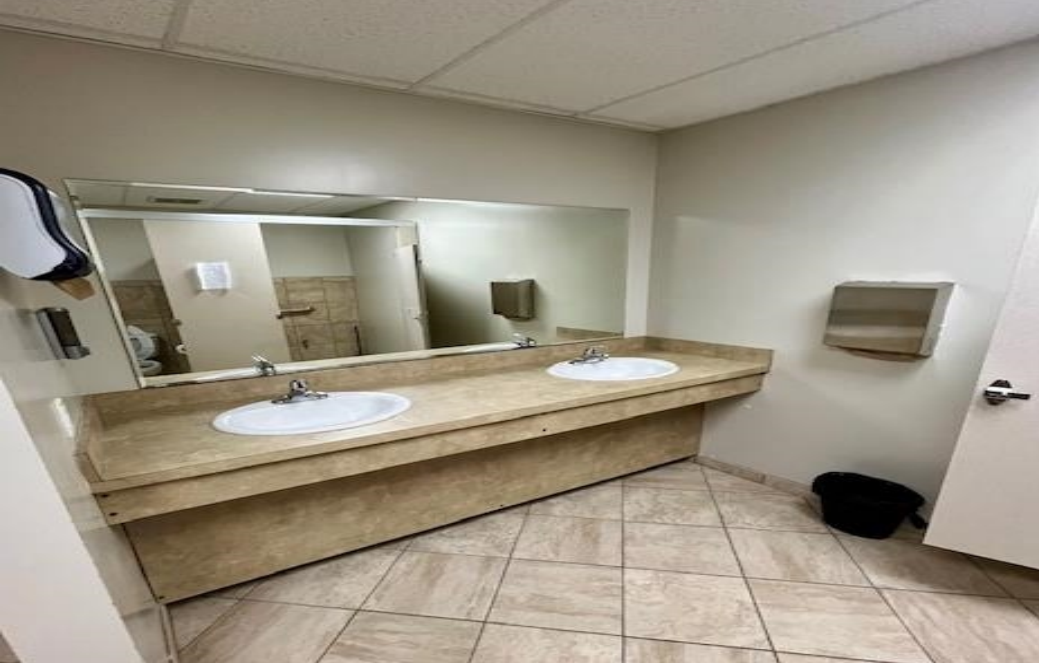
1st Floor Restroom
