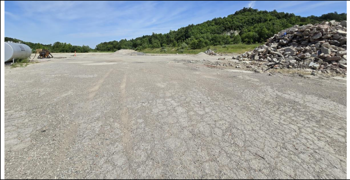
View of Subject Site
