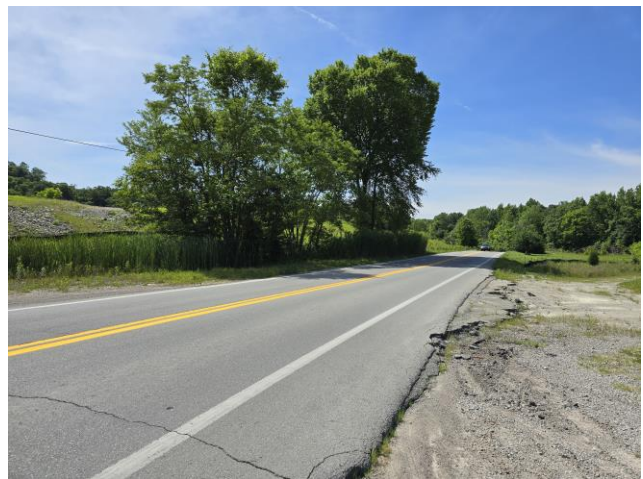
South Park Rd Facing East
