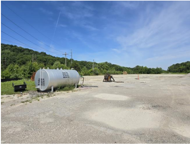
View of Subject Site
