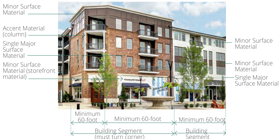
Figure 70.5.Q-1. Major and Minor Materials on a Facade
