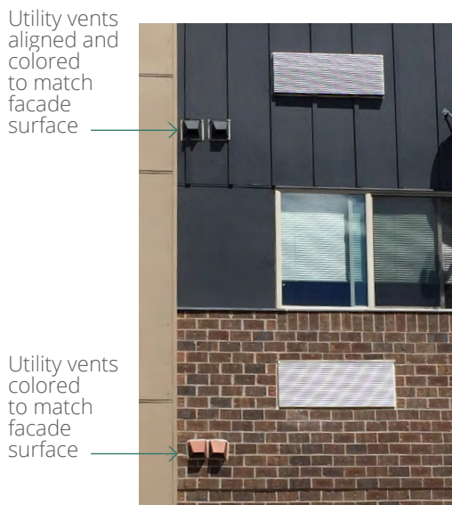
Figure 70.5.Q-16. Utility Appurtenances located on Facades
