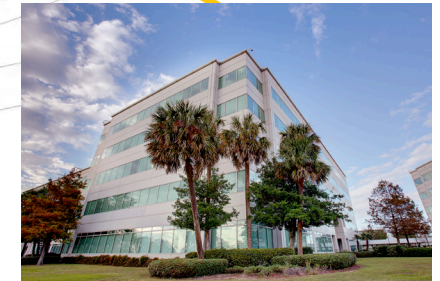
INFORMATION AND TECHNOLOGY CENTER #2 (ITC-2)
