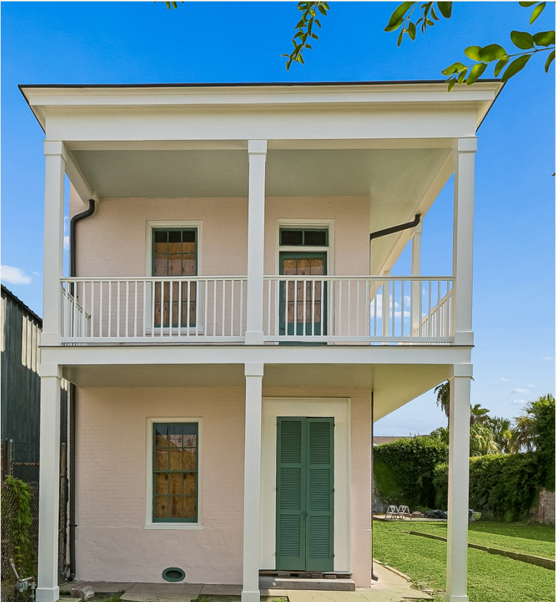
Existing Orange Street facade
