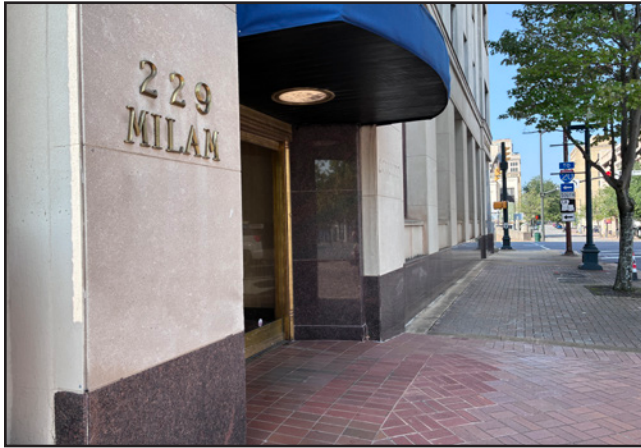
Side Entrance on Milam Street
