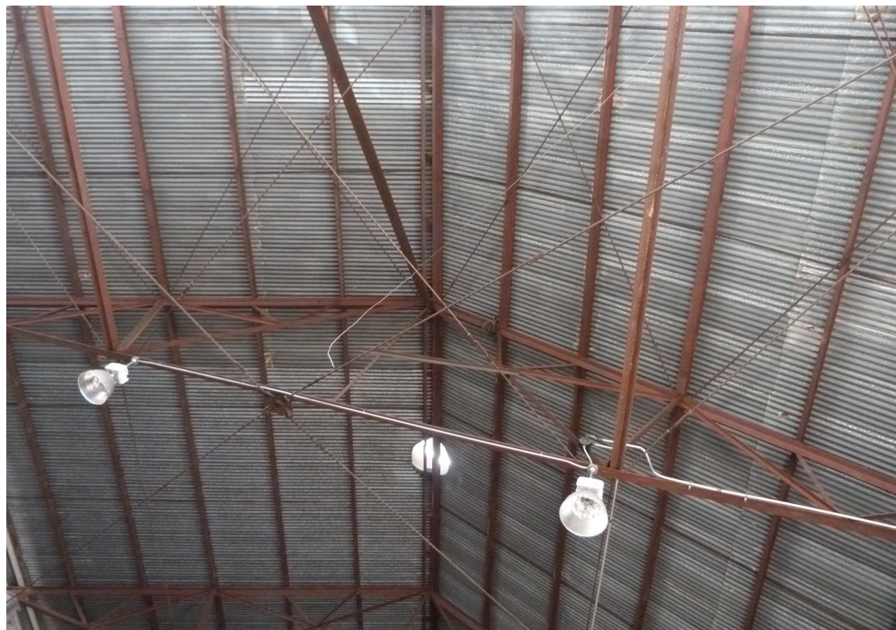
Existing steel roof structure and corrugated roof sheathing
