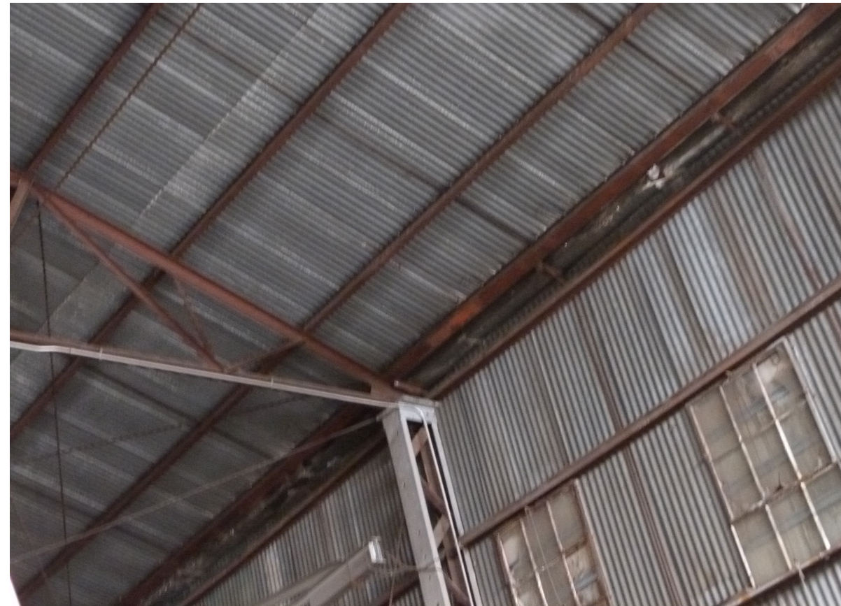
Existing roof and wall on Poeyfarre Street side: Corrugated metal
