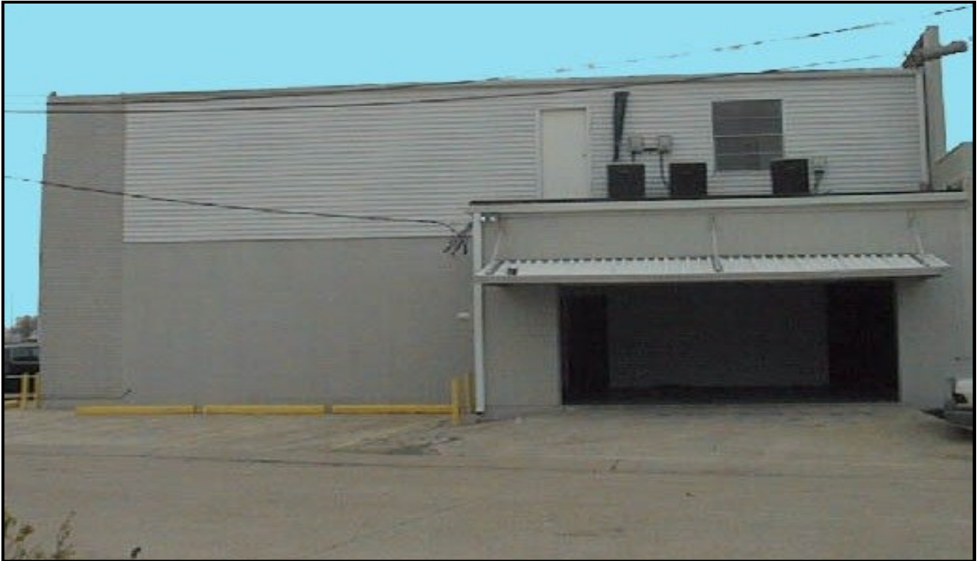
Warehouse Exterior Access
