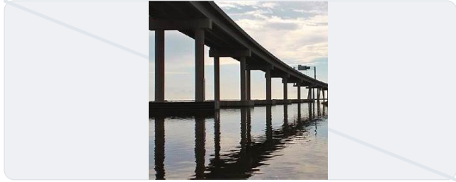
LA-1 Elevated Expressway
