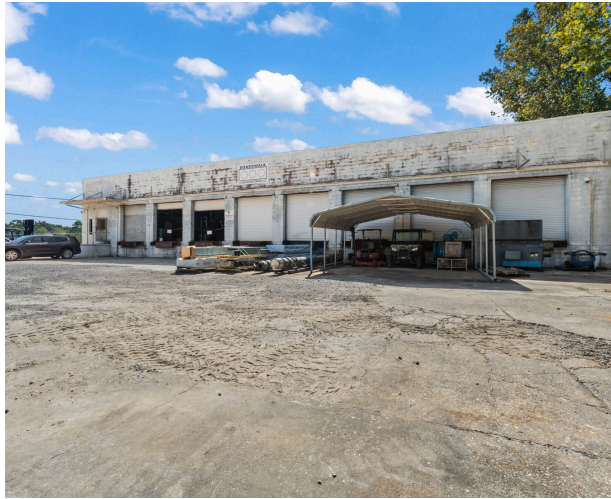
TRUCK APRON AND COVERED STORAGE
