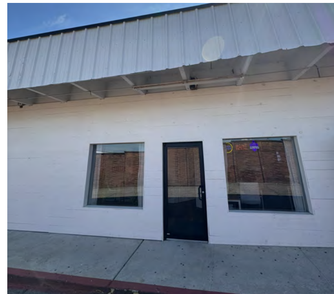
Suite D: Commissary Prep/Kitchen
