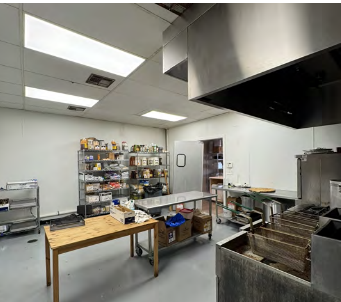
Suite D: Commissary Prep/Kitchen
