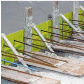
Formwork stop-end with continuity reinforcement
