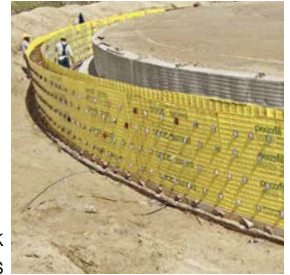
Circular formwork for foundations
