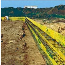
Installation of Pecafil® above ground
