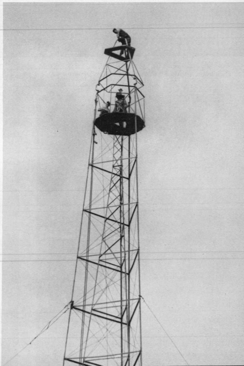
Final plumbing of tribrachs over pillar
