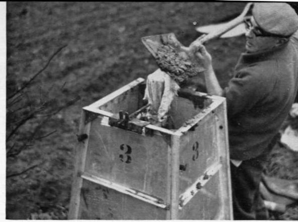
Filling the shuttering
