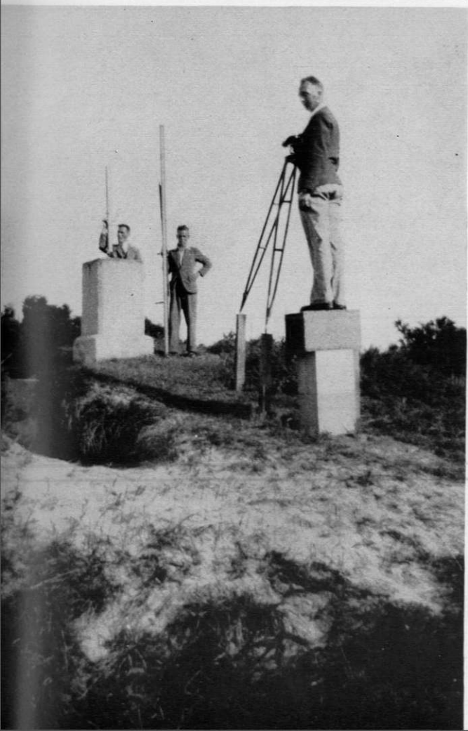
A difficult set-up for the levellers at the western terminal – a pillar erected for the 1910 measurement
