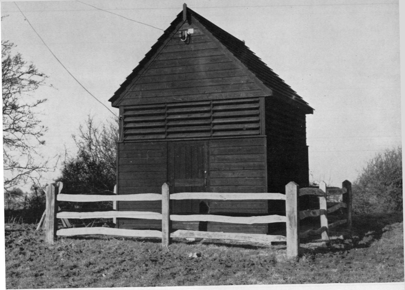
Exterior view of protecting hut, from south
