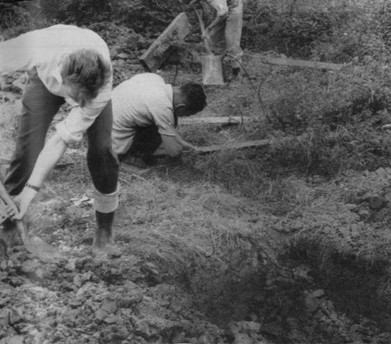
Excavating for footings
