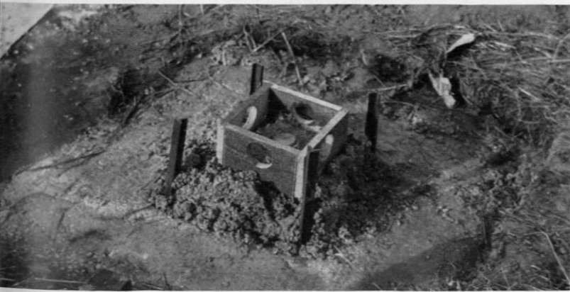
Top bolt, box, and angle-irons in position
