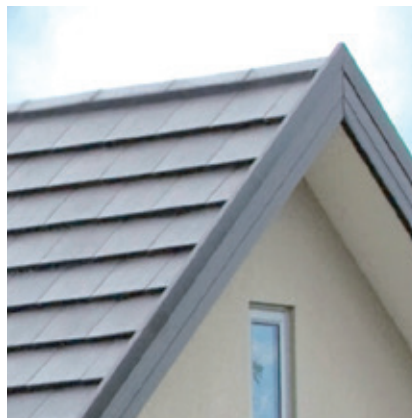
Gutter Barge finish
