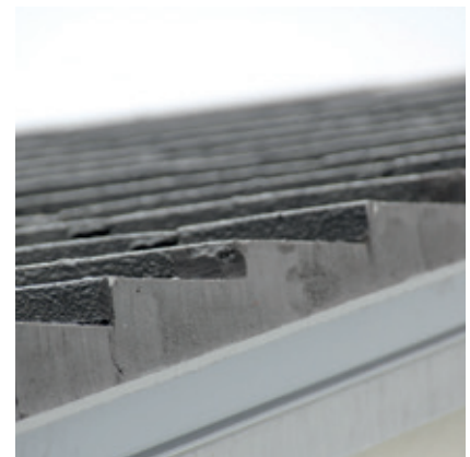
Bed and Point Barge finish
