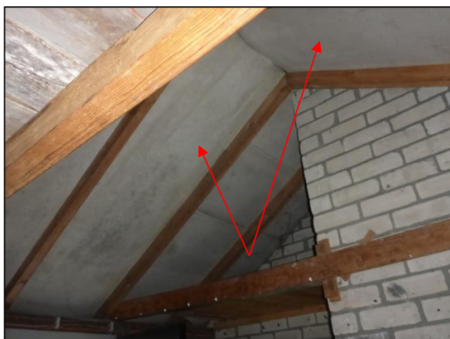
Foto 35: Berging: Dakbeschoot (Bron 3)
