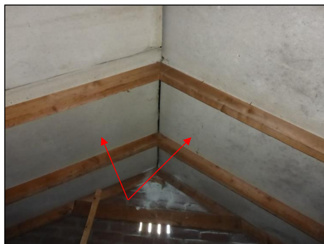
Foto 36: Berging: Dakbeschoot (Bron 3)
