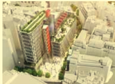
LSE's new social sciences centre has been designed by Rogers Stirk Harbour + Partners.
