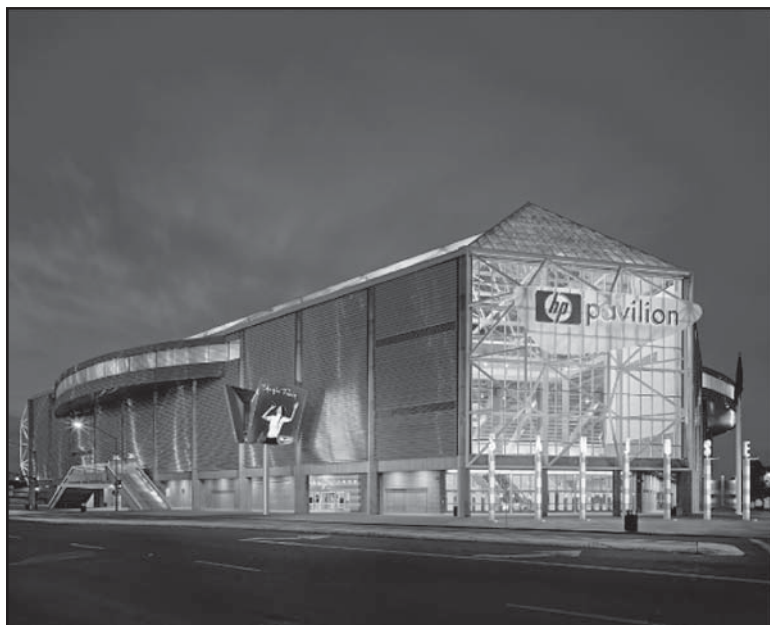
HP Pavilion - Home of the San Jose Sharks
